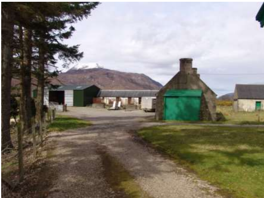
Kennels and associated buildings at the Keeper's House, Kinlochewe.
